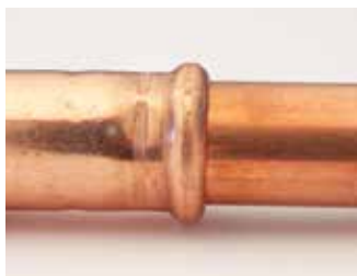
Pressed fitting - indents on the fitting.
