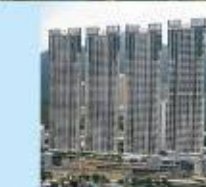
Phase 3, Festival City 盛世(名城3期) 1 Mei Tin Road, Tai Wai Developer: Cheung Kong Consultant: Parsons Brinckerhoff (Asia) Ltd. B.S. Contractor: Yuen Cheong Engineering Co., Ltd.
