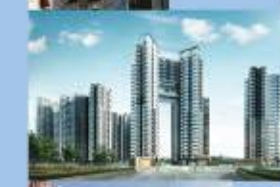
The Reach 尚悅 11 Shap Pat Heung Road, Yuen Long Developer: Henderson Land & New World Development Consultant: Meinhardt (M&E) Ltd. B.S. Contractor: Majestic Engineering Co., Ltd.
