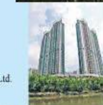
The River Park 漆岸8號 8 Che Kung Mui Road, Sha Tin Developer: New World Development & MTR Consultant: Parsons Brinckerhoff (Asia) Ltd. B.S. Contractor: Majestic Engineering Co., Ltd.
