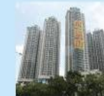
Lions Rise 現崇山 8 Muk Lun Street, Wong Tai Sin Developer: Kerry Properties Consultant: WSP B.S. Contractor: Yuen Cheong Engineering Co., Ltd.
