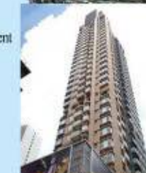
18 Upper East 港島·東18 18 Shing On Street, Shau Kei Wan Developer: Emperor Investment Consultant: Hyder Consultant Ltd. B.S. Contractor: Wong Kwong Kee Engineering Co., Ltd.
