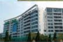
Providence Bay 天賦海灣 TPTL187 Pak Shek Kwok, Tai Po Developer: Sino Land, Nan Fung, K. Wah & Wing Tai Consultant: P & T Architects & Engineers Ltd. B.S. Contractor: Ridgid Plumbing Ltd.
