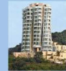
Opus Hong Kong 傲璇 53 Stubbs Road, The Peak Developer: Swire Properties Consultant: Parsons Brinckerhoff (Asia) Ltd. B.S. Contractor: ATAL Engineering Co., Ltd.
